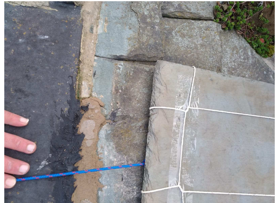
Proposed slate in place on roof- Vermont Green Slate
